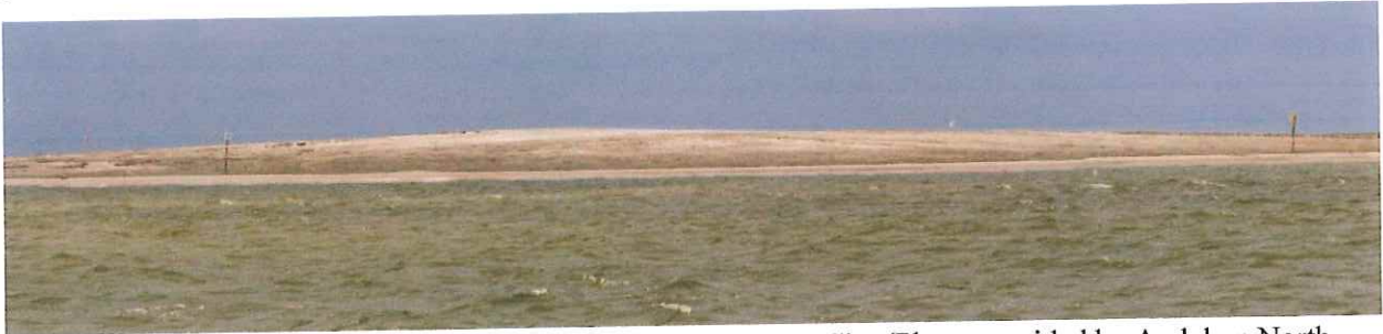
Figure 5. Post Construction Condition of Material Placement Site (Photo provided by Audubon North Carolina.)
